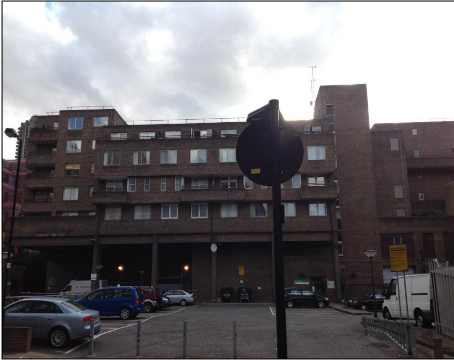
View of the rear of Shire House facing onto the application site from Lamb's Passage.
